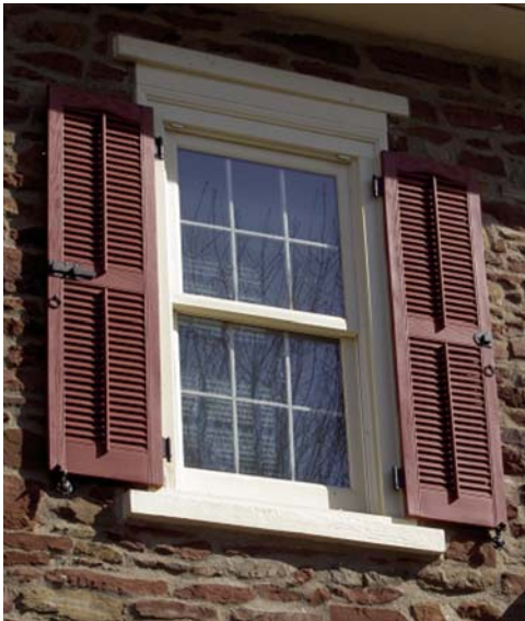
Vinyl shutters with Classic Accents hardware. The owner of this farmhouse added louver operators for authenticity.
